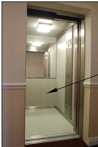
Photograph showing car walls
